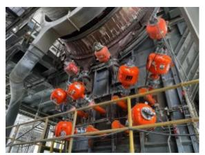
Air Cannons like Martin's Hurricane are in widespread use around the world in industries such as cement, steel, lime, coal, biomass, fertilizer and more. (Copyright © 2024 Martin Engineering)
