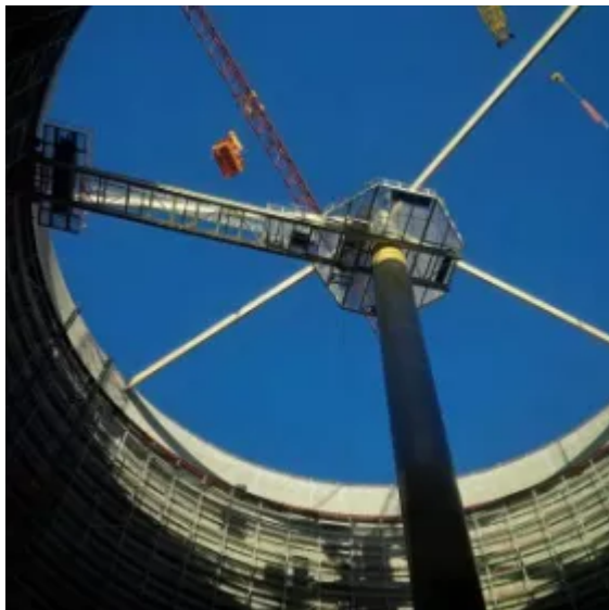
Installation of the starch silo equipment.
